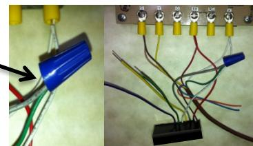
Connect the **Green** wire of the HVAC-CHIP to that "G" terminal. Note that only one wire is on this terminal. *This means that the HVAC-Chip's Green wire is now directly connected to the blower fan solenoid wire.*
