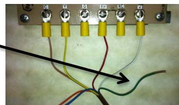
Add the **Brown** wire of the HVAC-CHIP to the existing wire at terminal “**C**” which is the 24V Common wire. This means 2 wires at this terminal when the connection is complete.
