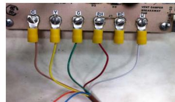
**STEP 4:** Take a photo or make a sketch of the wire connections. Make sure those connections are clear and readable. This will help if reconnection of original wiring becomes necessary.
